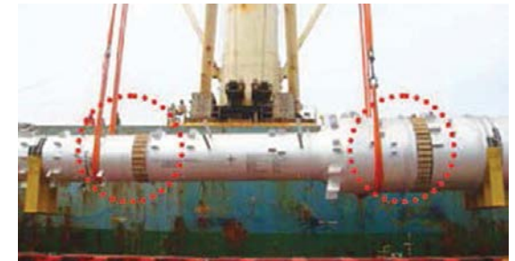
A single crane lifts a column horizontally. The position of the slings here, offset from wooden battens, indicate an off-centre CoG.
